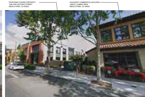
(C) RIGHT SIDE PROPERTY AND ADJACENT COMMERCIAL BUILDING VIEW
