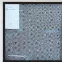
POSITIVE FRIT PATTERN FOR GLARE REDUCTION
