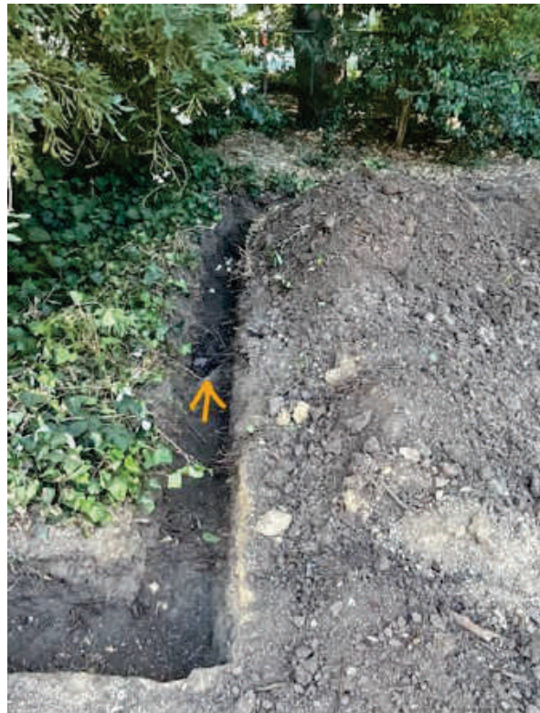
Photo 2 – one root from tree #23, arch or bridge over
