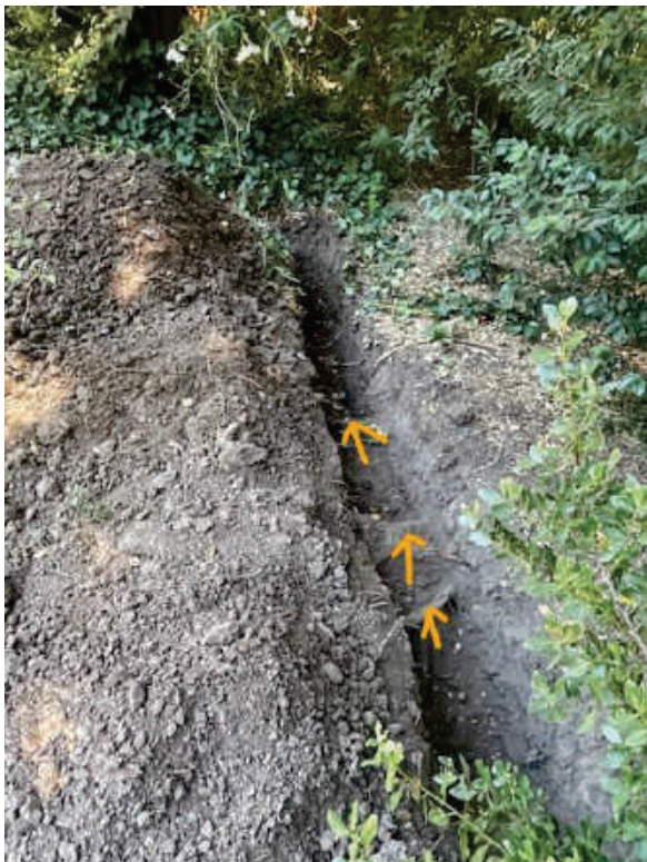
Photo 3 – three roots from tree #23, 2 lower to arch or bridge over, 1 higher to space around for pour
