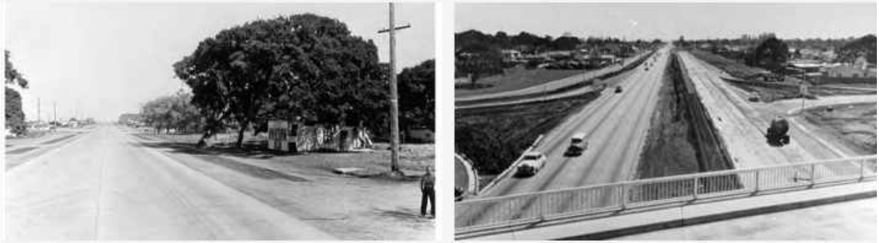
Figure 2. Highway 101 Divides the Community, Before and After Widening
