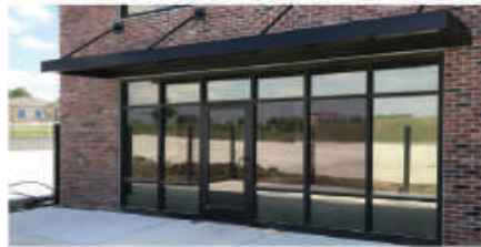
W2 STOREFRONT ALUMINIUM STOREFRONT BLACK FRAME FINISH
