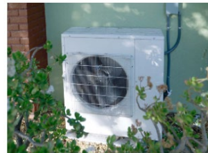
Heat pump condenser evaporator unit
