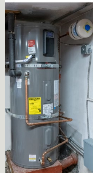
Installed heat pump water heater
