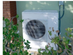
Heat pump condenser evaporator unit
