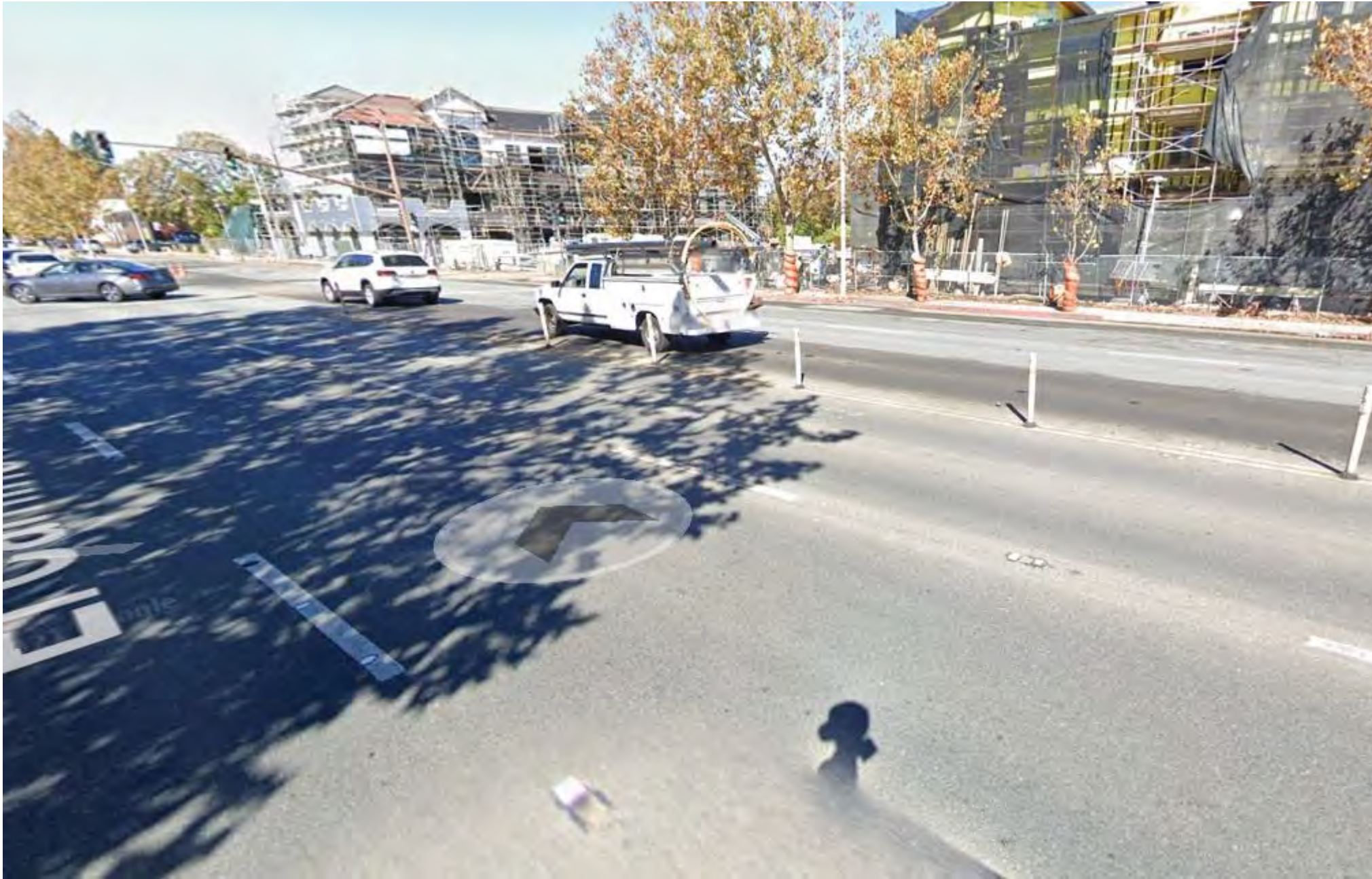
EXISTING STRIPED MEDIAN ISLAND WITH FLEXIBLE VERTICAL POSTS
