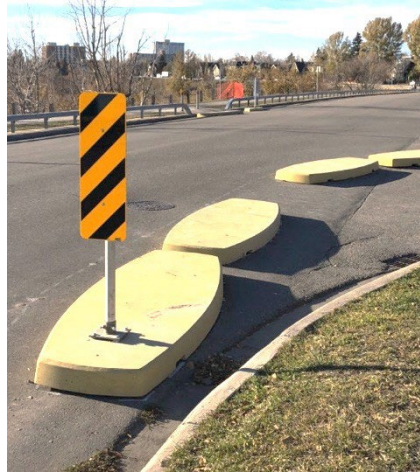
(Temporary Traffic Calming Curbs, Calgary, AB)
