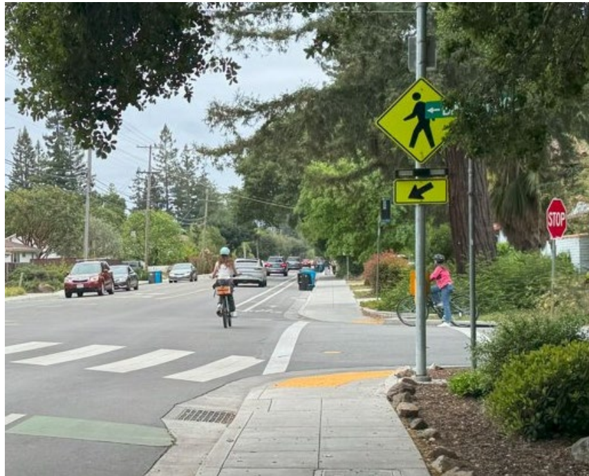
Figure 5-16: Trees Blocking Street Sign
