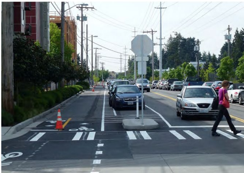
Figure 5-17: Existing One-Way Bike Lane
