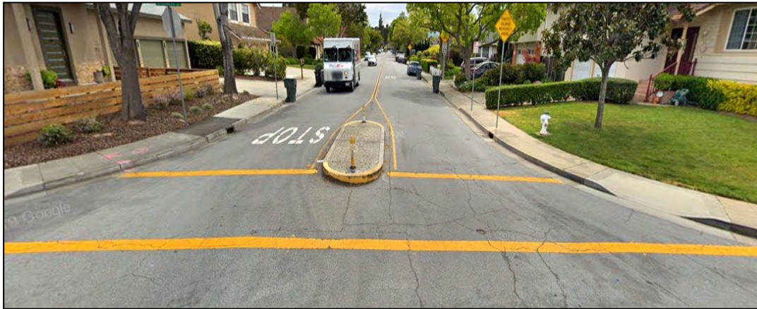
Figure 5-5: Median Island on Residential Street
