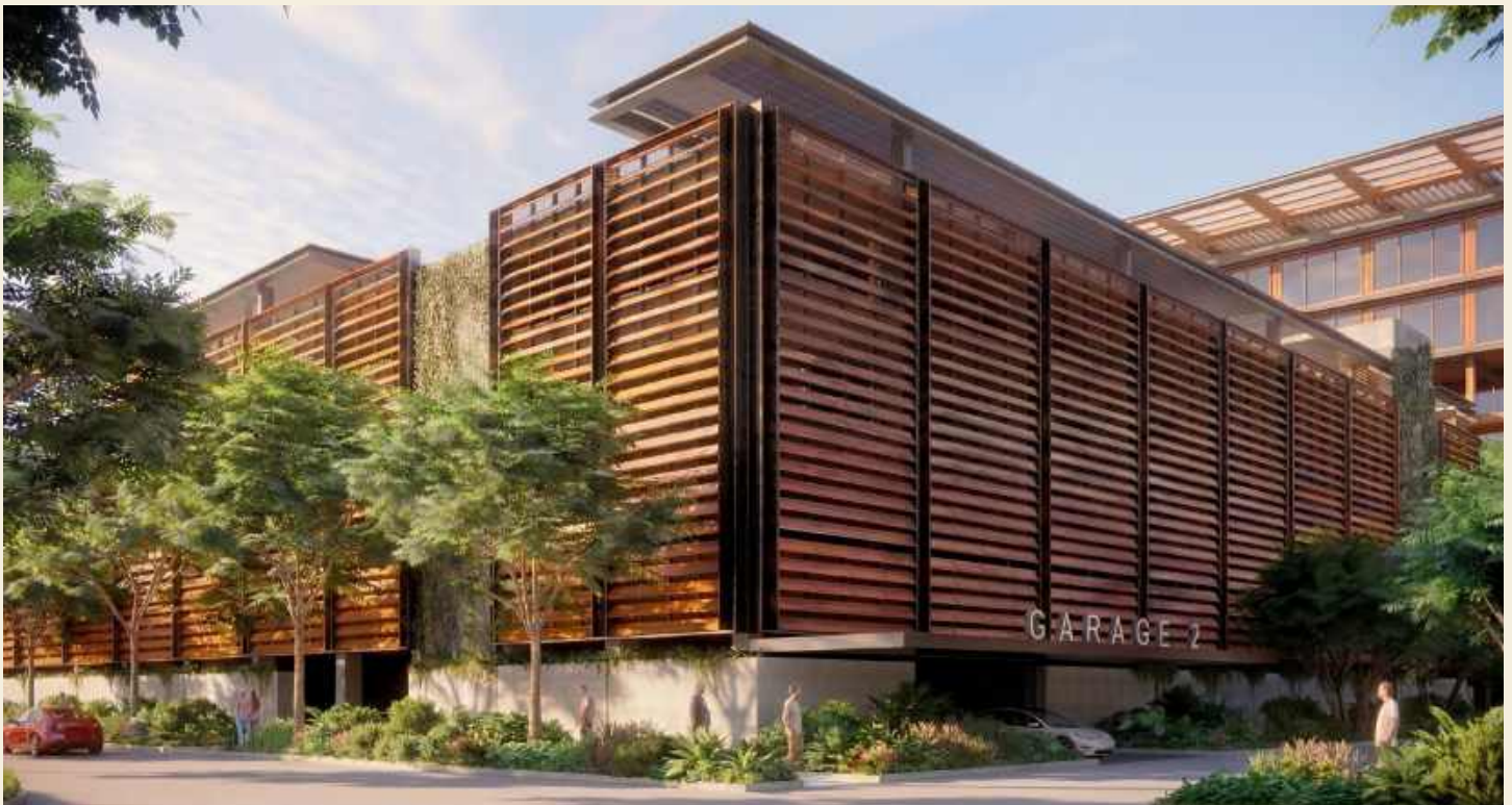
View of Parking Garage 2 from the entry off Middlefield Road
