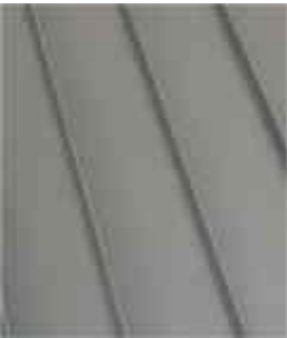
2 2NDING SEAM METAL ROOF
