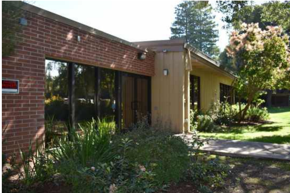
Figure 8: West end of south façade, view northeast.
