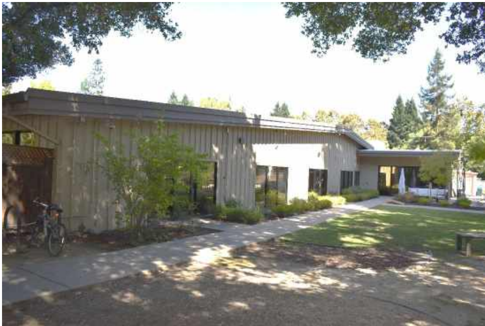
Figure 10: South end of east façade, view northwest.
