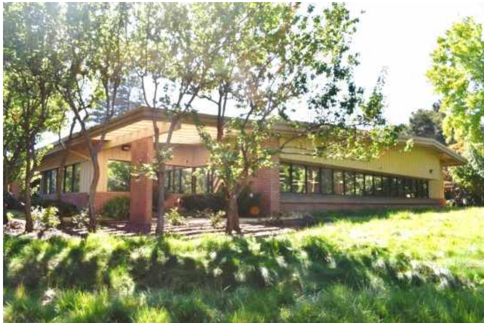
Figure 5: North end and center of the west façade, view southwest.
