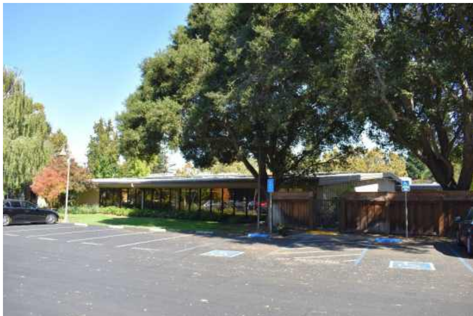
Figure 9: East end of south façade, view northwest.
