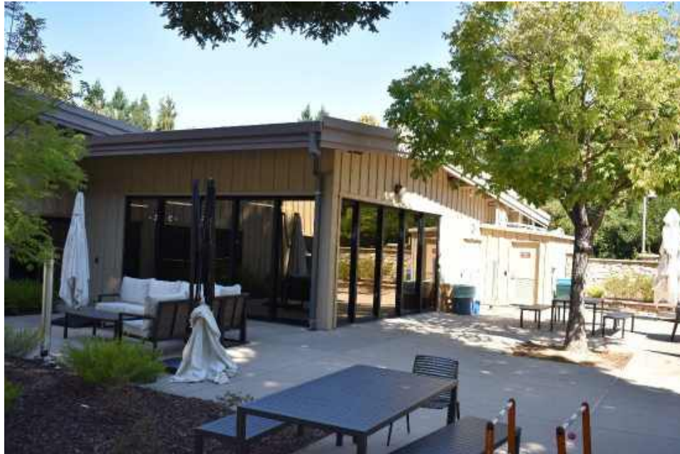
Figure 11: North end of east façade, view northwest.
