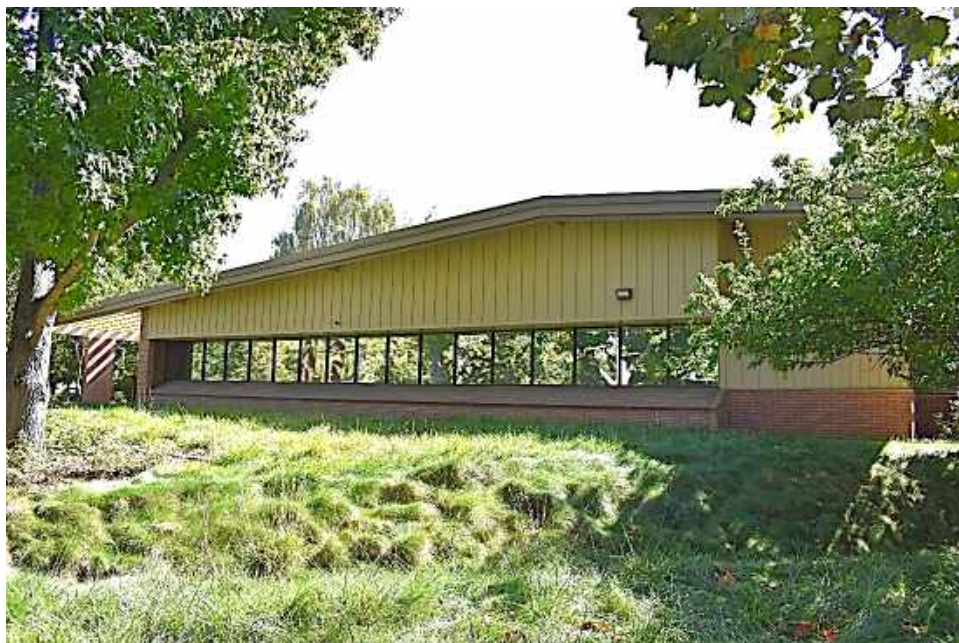
Figure 6: North end and center of west façade, view northeast.
