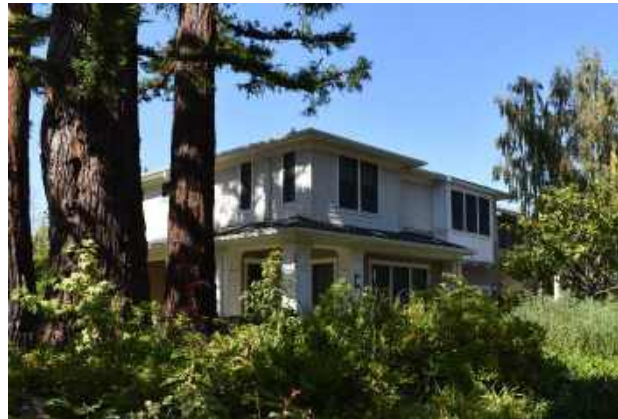
Figure 19: 841 Paulson Circle, single family house built 2008.
