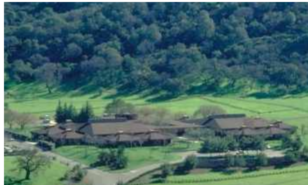
Figure 26: IBM Los Gatos Laboratory (1964, since demolished) in San Jose, designed by Hellmuth, Obata, & Kassabaum. Source: HOK.
