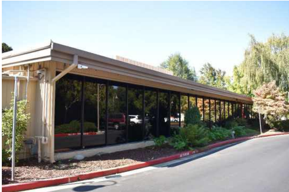
Figure 3: East end of the primary (north) façade, view northwest.
