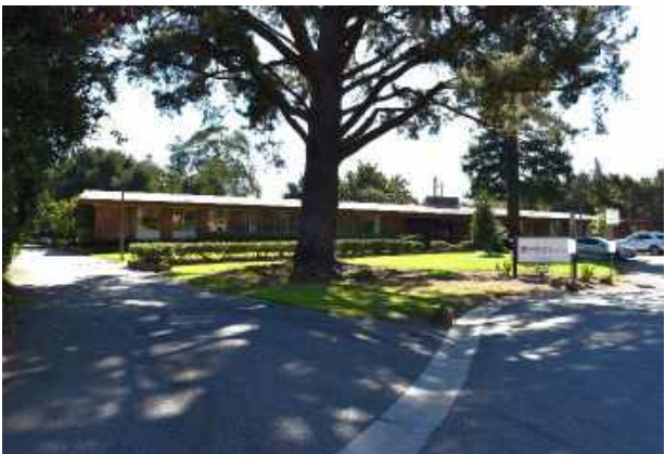
Figure 20: 66 Willow Place, office building built ca. 1955.
