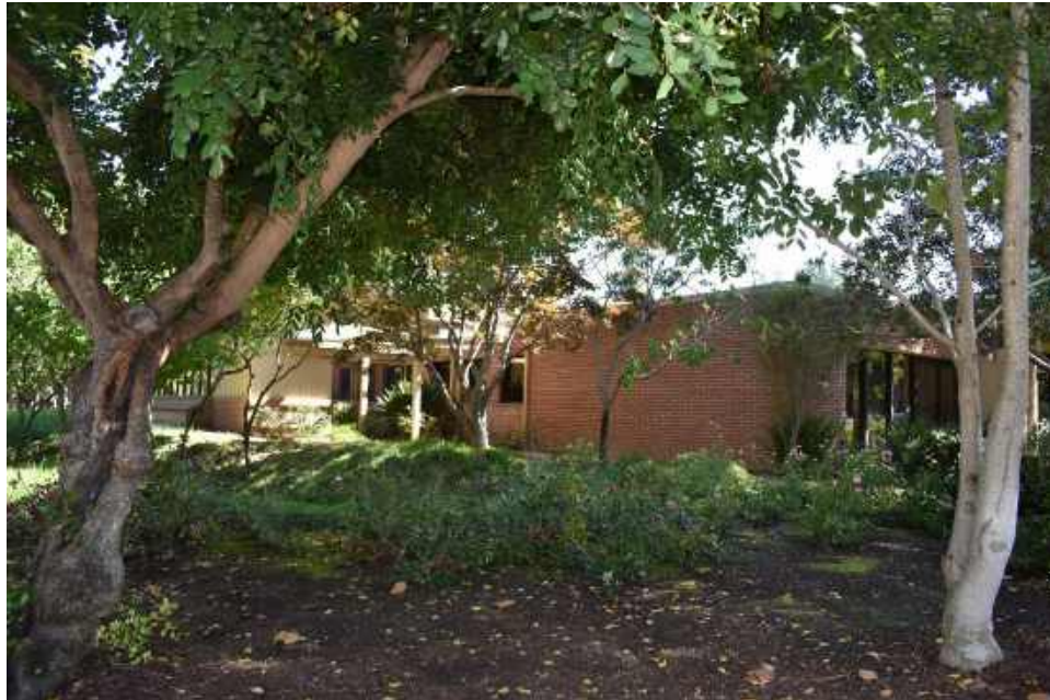
Figure 7: South end of west façade, view northeast.
