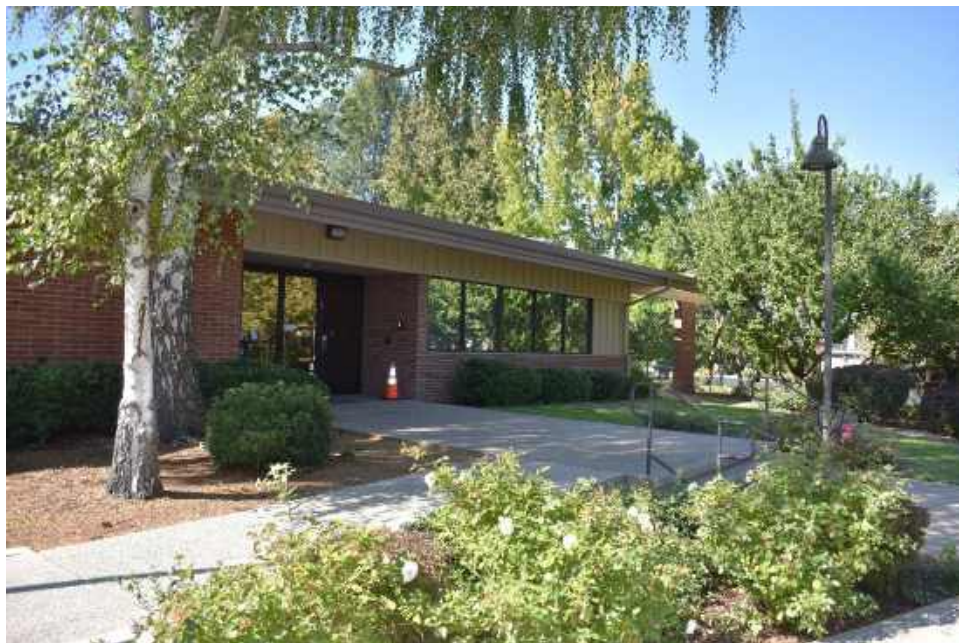
Figure 4: West end of the primary (north) façade, view northwest.
