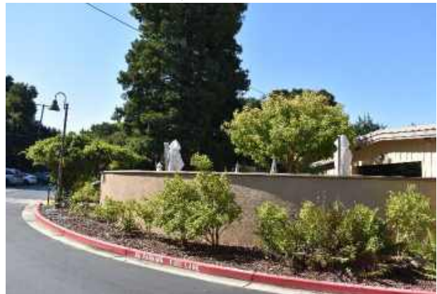
Figure 15: Site wall at northeast corner of site, view southwest.
