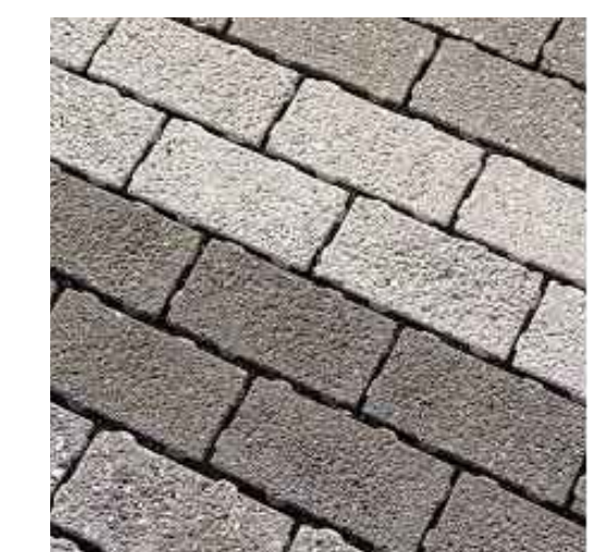
① PERMEABLE UNIT PAVERS
