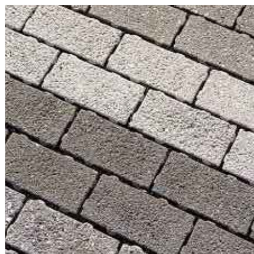
① PERMEABLE UNIT PAVERS
