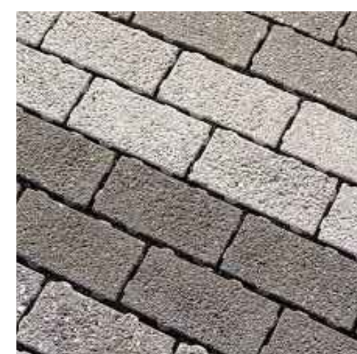
① PERMEABLE UNIT PAVERS
