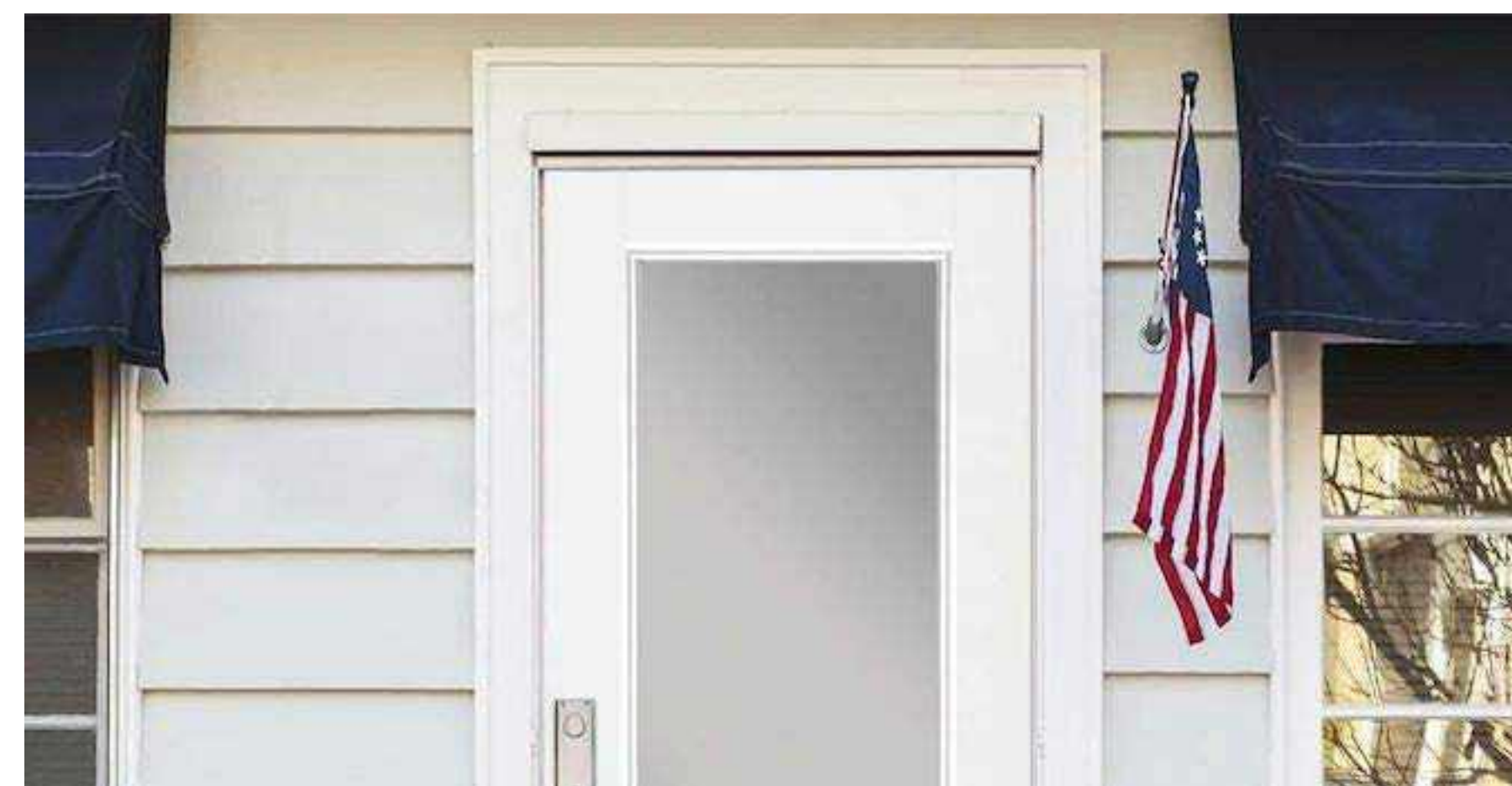
D - ENTRY DOORS - MASTERCRAFT FROSTED PRIMED STEEL DOOR OR EQ, COLOR WHITE
