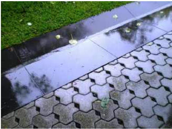
Sustainable design of parking lot using permeable surfaces (Baltimore, Maryland)
