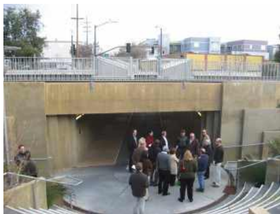
Pedestrian/bicycle tunnel linkage (Palo Alto, California)
