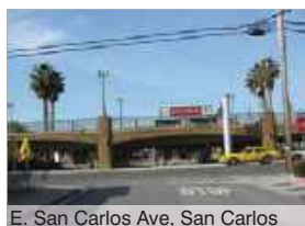
E. San Carlos Ave, San Carlos Underpass crossing in San Carlos (raised rail line)
