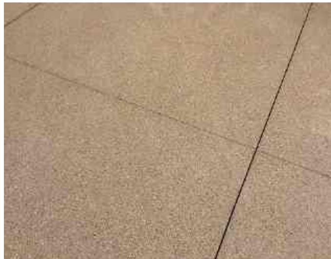
2 Enhanced Concrete Paving 3,750 Square Feet
