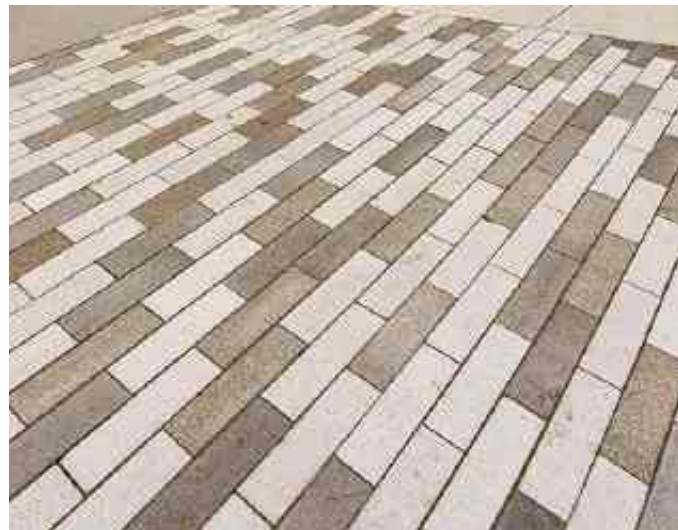
3 Concrete Pavers 2,400 Square Feet
