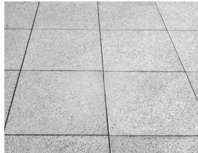
1 Standard Concrete Paving Existing To Remain Or Repair
