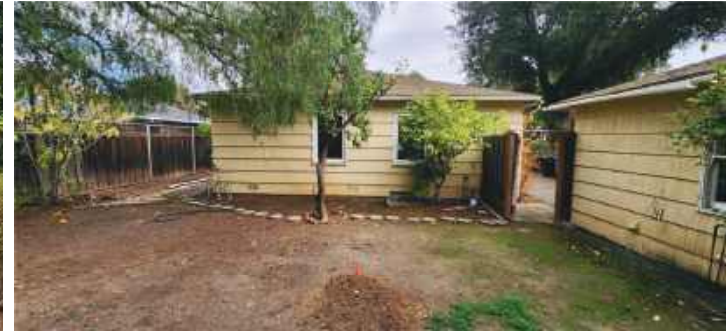
EXISTING MAIN STRUCTURE: WEST ELEVATION (REAR)
