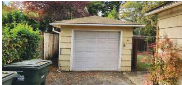
EXISTING ACCESSORY STRUCTURE: EAST ELEVATION (FRONT)
