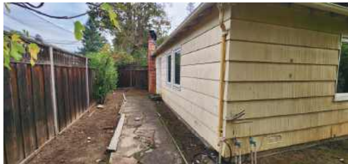
EXISTING MAIN STRUCTURE: NORTH ELEVATION (RIGHT SIDE)
