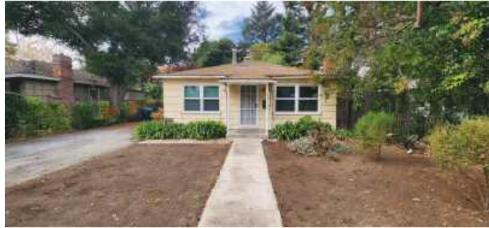
EXISTING MAIN STRUCTURE: EAST ELEVATION (FRONT)
