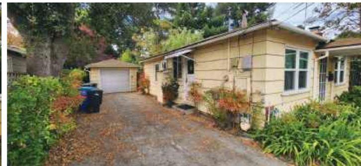
EXISTING MAIN STRUCTURE: SOUTH ELEVATION (LEFT SIDE)
