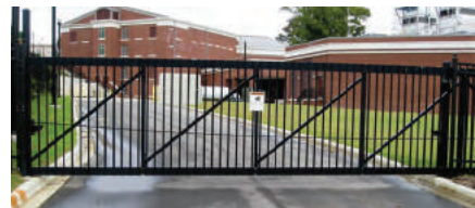
3 6-FOOT HIGH SLIDING GATE SCALE: N/A
