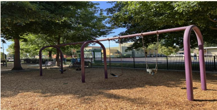
Swing set 2 belt, 2 infant — chipped paint over rust
