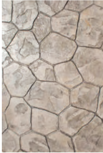
PAVEMENT NODE - STAMPED CONCRETE
