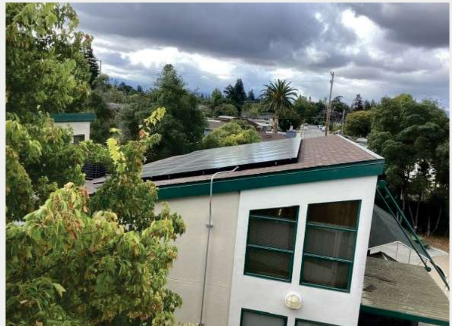
Newly installed solar on the roof of the BHCDC
