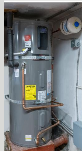
Installed heat pump water heater
