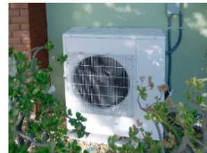
Heat pump condenser evaporator unit
