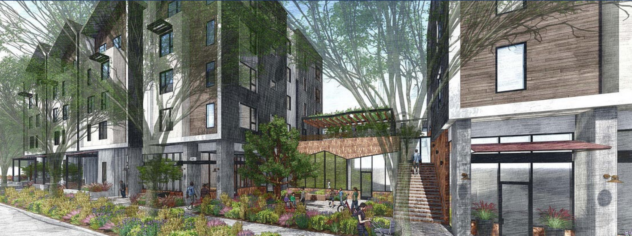
Corso (Mountain View Lot 12): 120 Affordable homes under construction by Related and Alta
