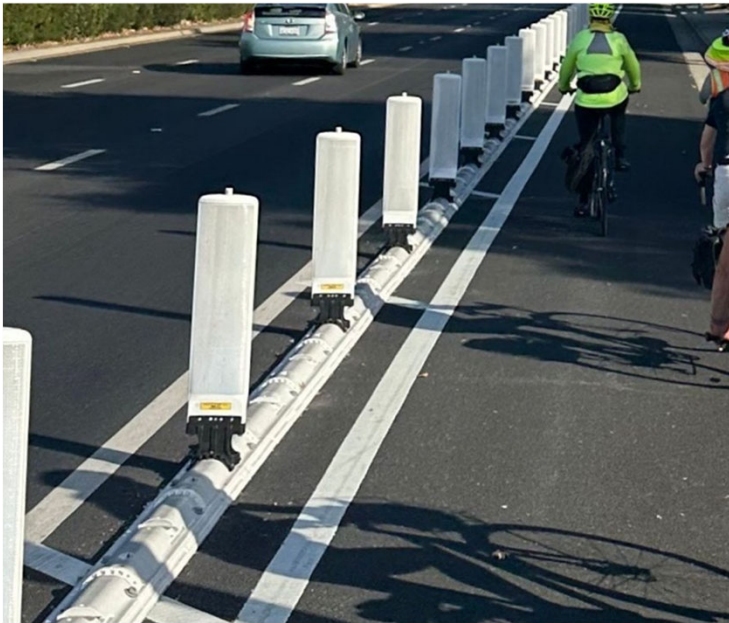
Curb-and-post separators on the El Camino Real bikeway: posts on a low curb base. Detail from Complete Streets Commission packet, Aug. 27, 2026, Att. D-1
