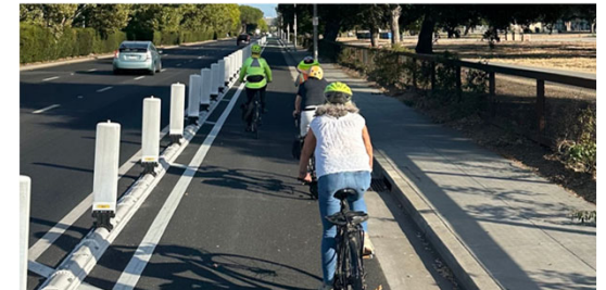
Riders behind flexible posts on El Camino Real. Complete Streets Commission packet, Aug. 27, 2026, Att. D-1
