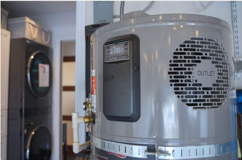
Heat pump water heater
