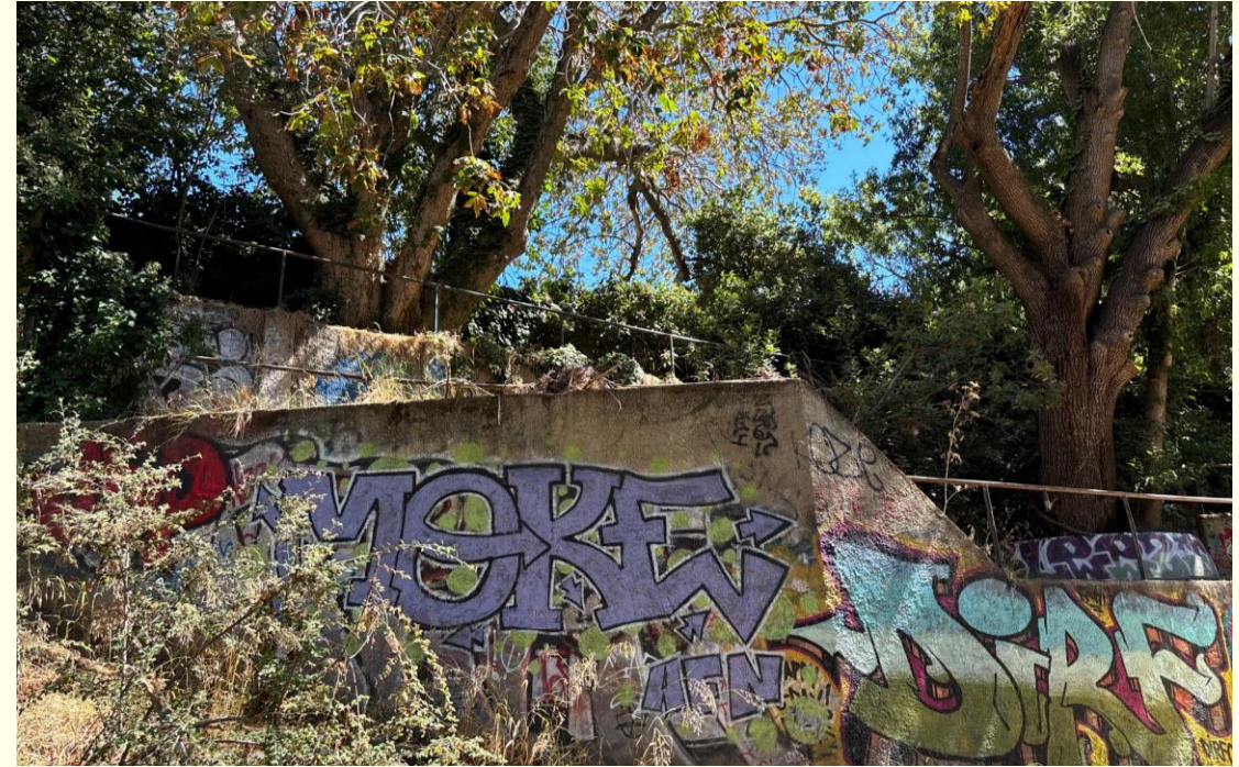
Picture of a concrete structure creating a pinch point that would be removed during channel widening
