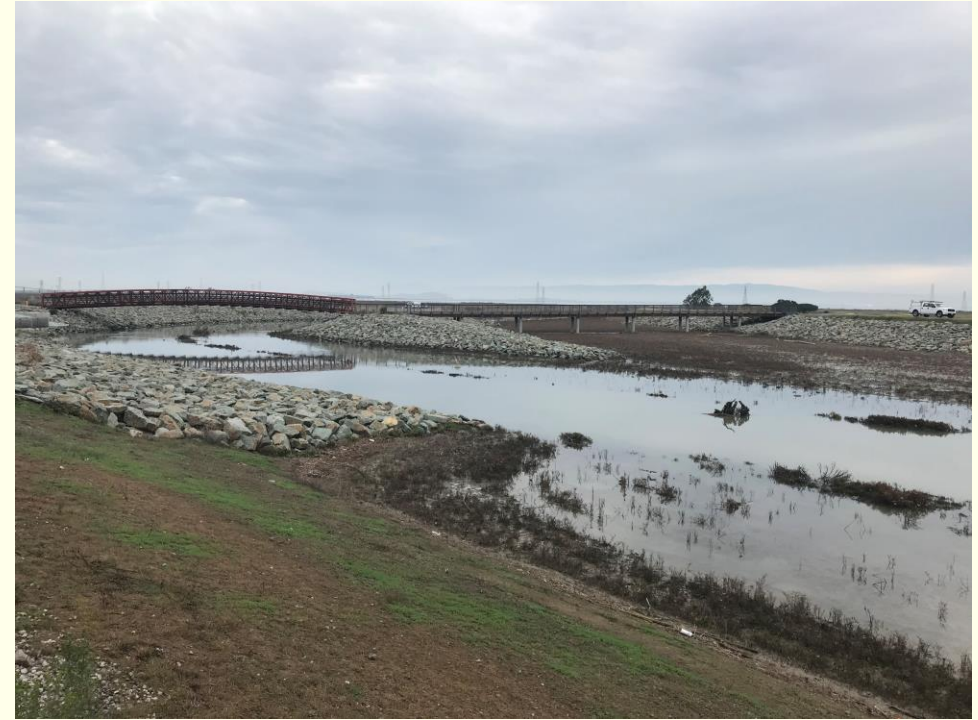
Completed Reach 1 Project at Friendship Bridge
