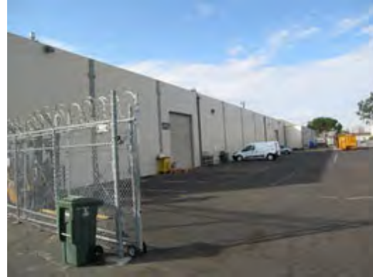
Rear (Easterly Elevation) of 985 O'Brien Drive
