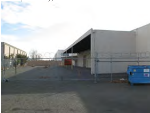
Rear (Easterly) Elevation of 1001 O'Brien Drive
