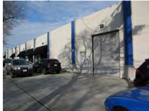
Front (Westerly) Elevation of 1001 O'Brien Drive
