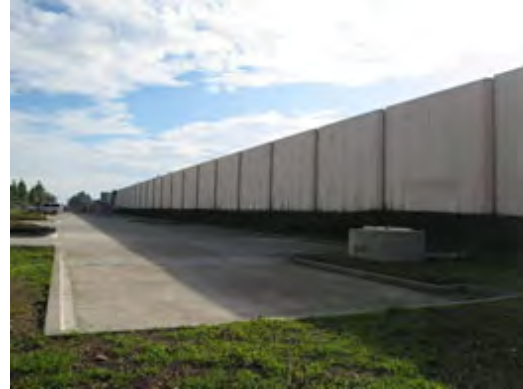
Rear (Easterly) Elevation of 1320 Willow Road
