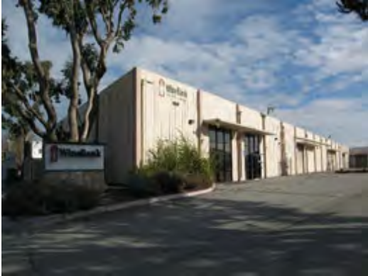
Front View of 1320 Willow Road
